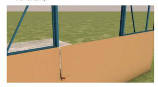
2. Cut *Kingspan* **AIR-CELL®** carefully around doors, windows and other openings, so that it neatly abuts to frames.
