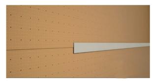
3. Butt join *Kingspan* **AIR-CELL®** sheets and tape with a 48 mm wide reinforced foil tape.
