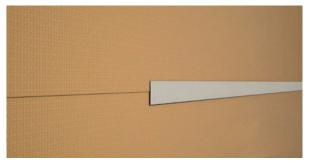
3. Butt join *Kingspan* **AIR-CELL** Insulshed<sup>®</sup> 50 sheets and tape with a 72 mm wide reinforced foil tape.
