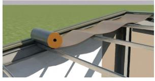
1. Lay *Kingspan* **AIR-CELL** Insulshed<sup>®</sup> 50 perpendicular to purlins ensuring a 25 mm overlap into the gutter.
