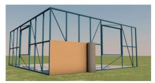
1. Fix *Kingspan* **AIR-CELL** Insulshed<sup>®</sup> 50 loosely to the outside of frame leaving flexibility for the insulation to be dished onto the wall cavity.
