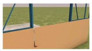
Cut Kingspan AIR-CELL Insulshed<sup>®</sup> 50 carefully around doors, windows and other openings, so that it neatly abuts to frames.
