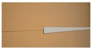
3. Butt join Kingspan AIR-CELL sheets and tape with a 48 mm wide reinforced foil tape.
