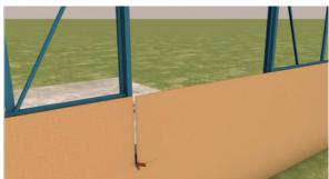
Cut Kingspan AIR-CELL carefully around doors, windows and other openings, so that it neatly abuts to frames.
